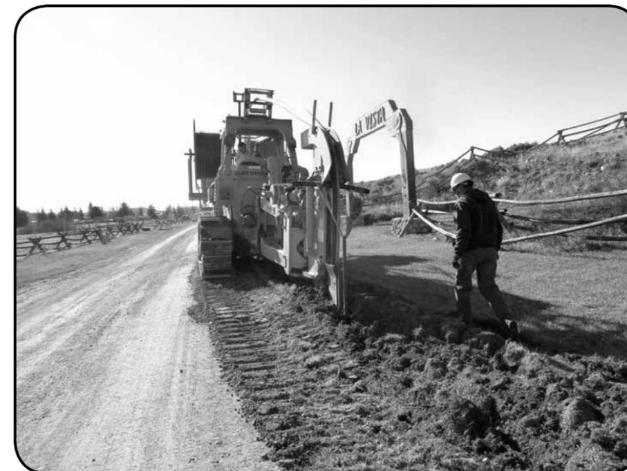
Dubois area foreman, Doug Cooley, supervises as new power and communications cables are installed at Stoney Point as part of a system upgrade. The original high voltage direct burial cable has come to the end of its serviceable life and is being replaced with a better insulated jacketed cable in conduit which should result in a much longer life span.
