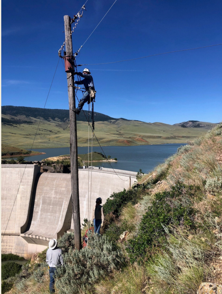
THERMOPOLIS CREW PUTTING UP NEW POLE AND TRANSFORMER AT ANCHOR DAM.
