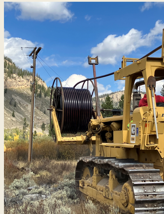
DUBOIS CREW WORKING ON A PLOW JOB AND LAYING CABLE.
