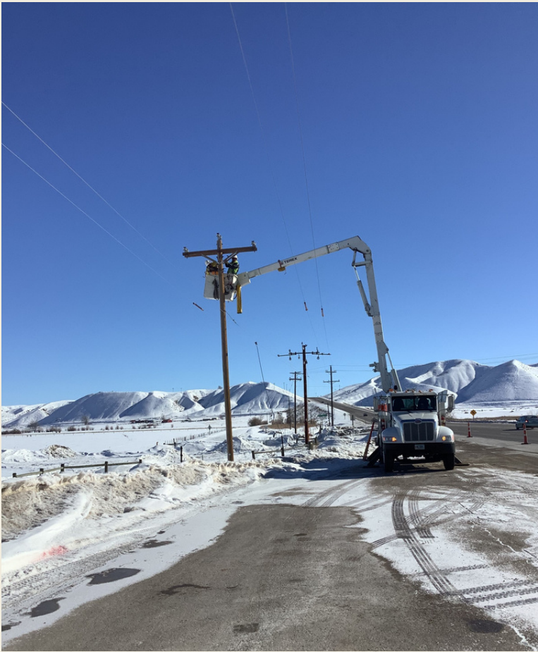
Photo credit: JD Watson, Crossarm Replacement Hudson/Lander
