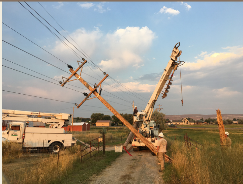
Photo credit: Brian Heiner, Pole replacement after windstorm
