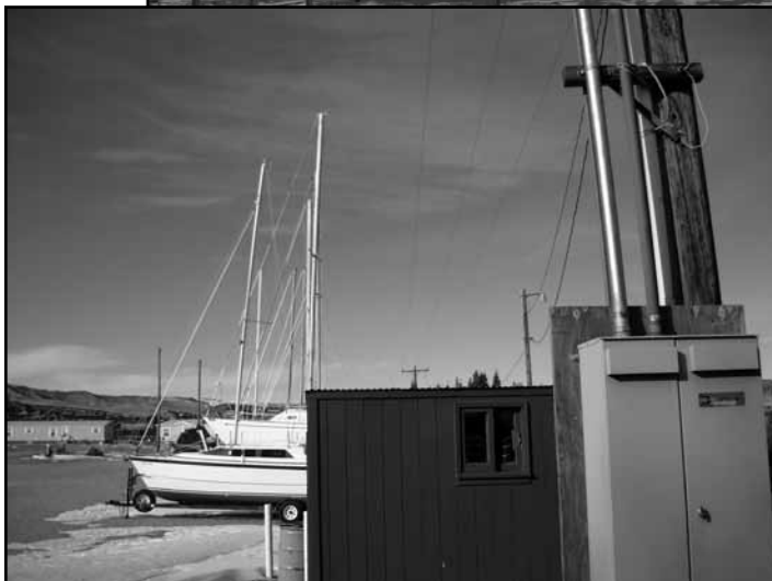
Left: These sailboats are entirely too close to a high voltage line. The steel rigging lines pose an extreme electrocution hazard.
