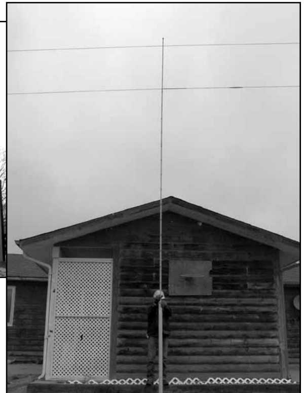
Above: Here is an example of an addition to a home that lacks proper, safe clearance from the power lines.
