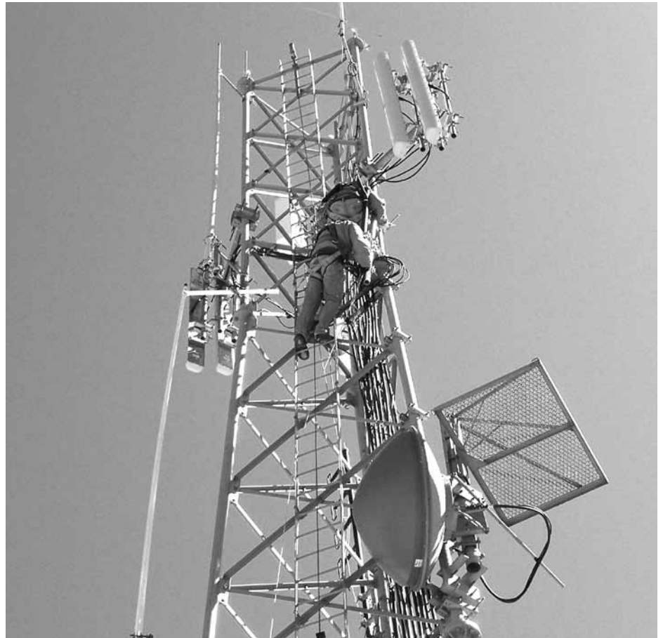
Contract communication technicians are attaching an additional antenna to a tower on Windy Mountain serving the Dubois area.
