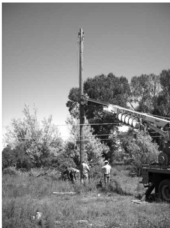
Beginning construction of the new 4-pole dead end structure
