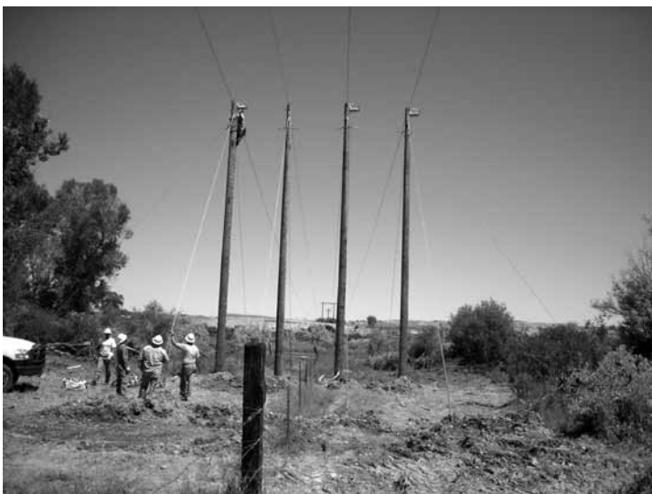
Completed construction of the structure
