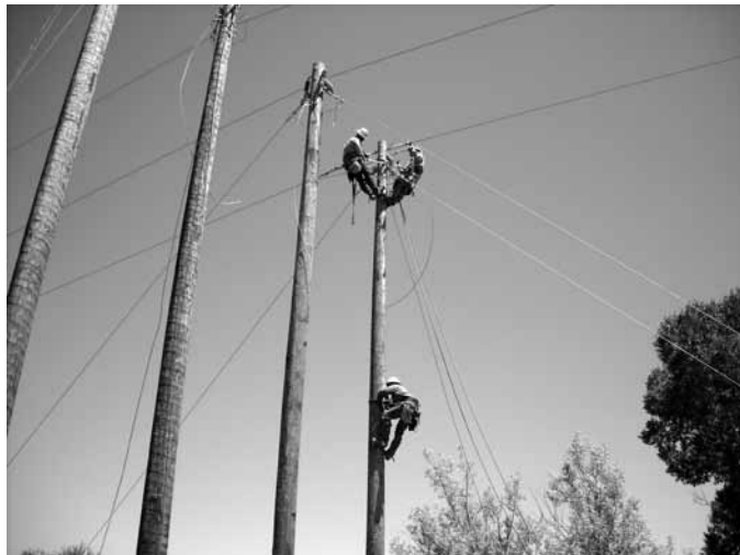
Ensuring correct tension on wire
