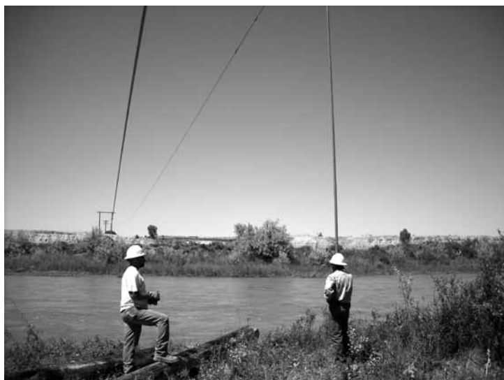
Measuring clearance at river bank
