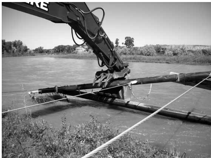
Downed structure being removed from the Wind River
